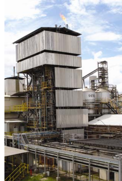
Image courtesy of Petrobras
