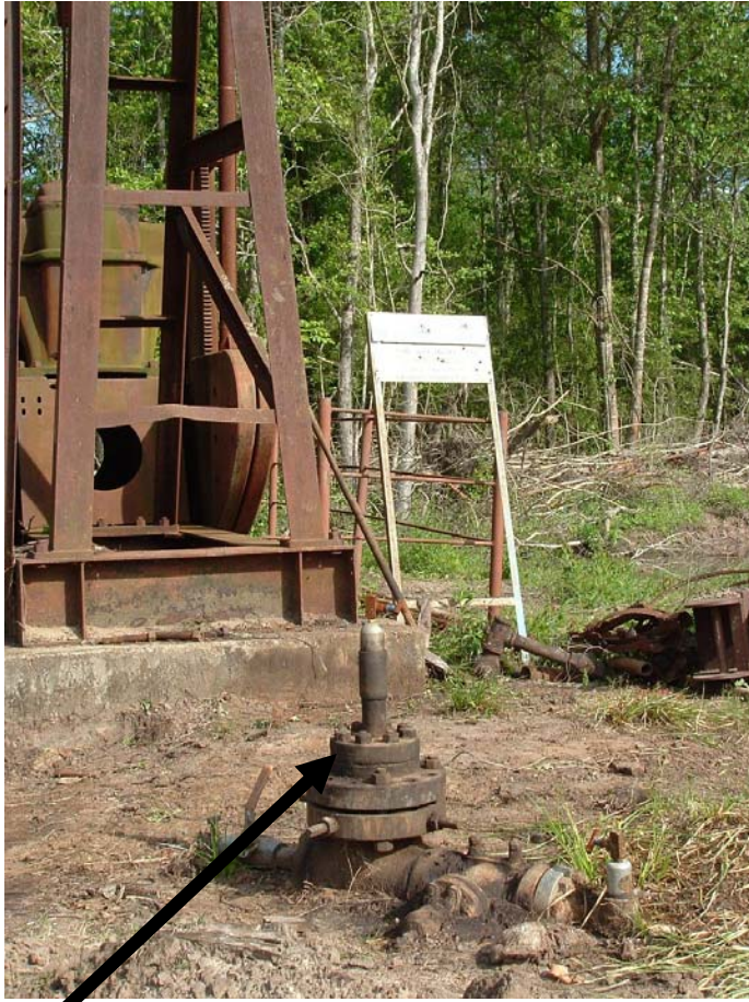
1952 oil production well was retrofit as an observation well
